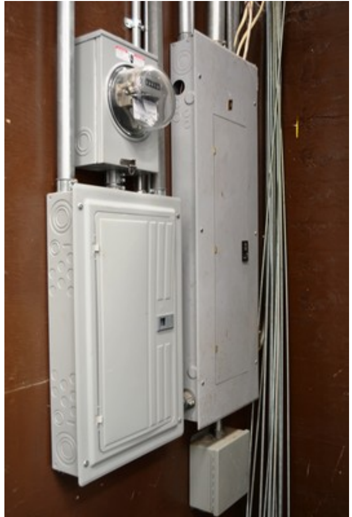
2-3phase panels, 200 amp and also 1 single phase panel 200amp
